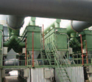
DELTAflex – modular system for 320,000 m³/h air flow
